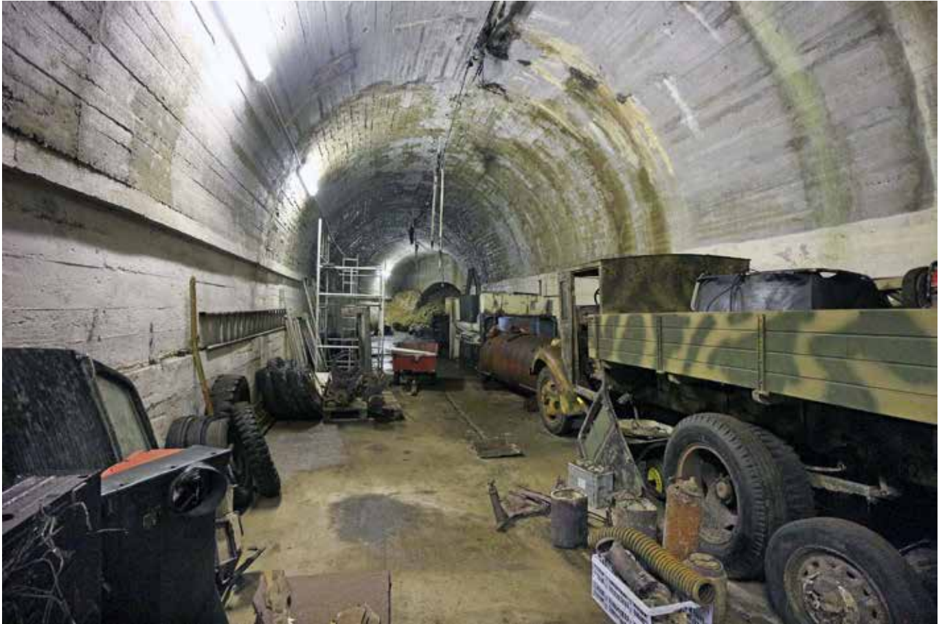
The southern access tunnel at Ho 1 is now used as a workshop by Festung Guernsey for the restoration of large and small items left behind by the Germans
